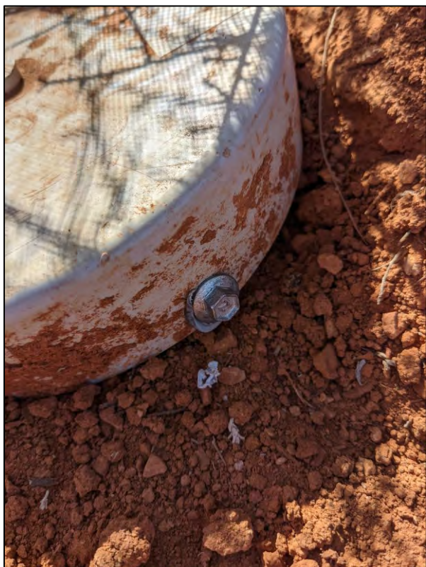
Figure 5. Tech-screws installed into pitfall lid at one of the flood-prone sites at conclusion of the survey.
