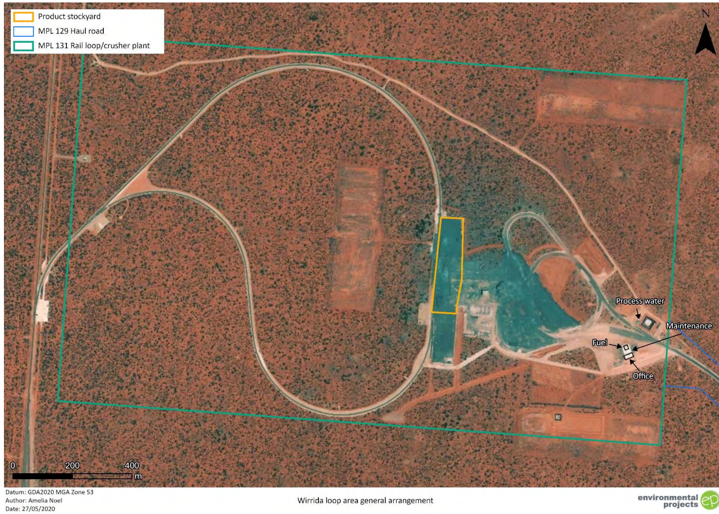
Figure 3-73: Rail loop facility
